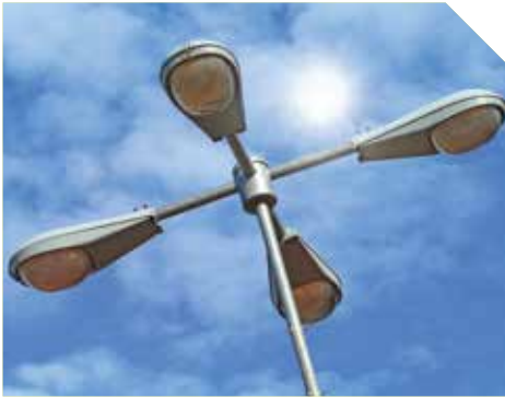
Swaged pole used at street lighting
