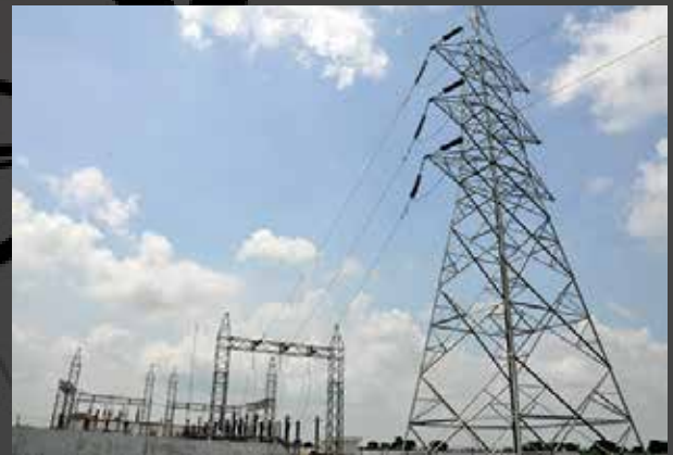
400 KV M/C Towers of Panchkula - Patiala T/L Project
