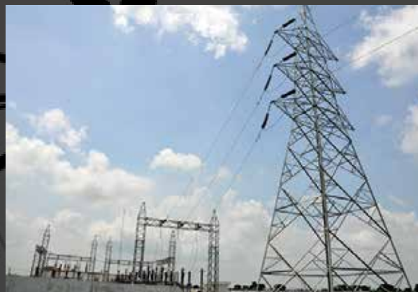
400 KV M/C Towers of Panchkula - Patiala T/L Project
